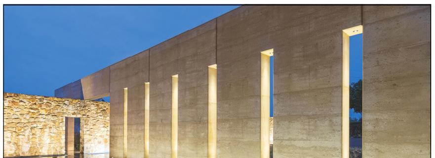
**COST EFFECTIVE:** Unlike other masonry, rammed earth walls don't need core filling or reinforcing. They are solid right through. Nor do they need plastering or painting, saving costs when you build – and for years. The walls won't get dented or marked and need repainting or touching up over the years to come. Once they're up, they're finished.
